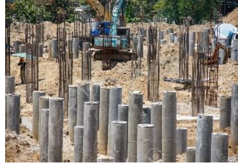
Figure 20. Deep foundations (pile foundations)
