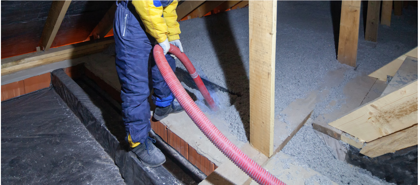
Attic insulation using cellulose wadding
