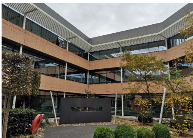
Façade of the Suravenir building in Brest, with sun-breaking blade caps
